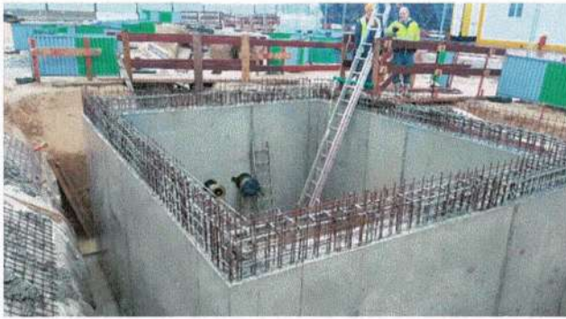
Construction of low point valves chamber
