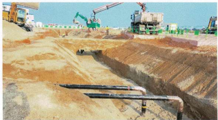
Backfill phase
