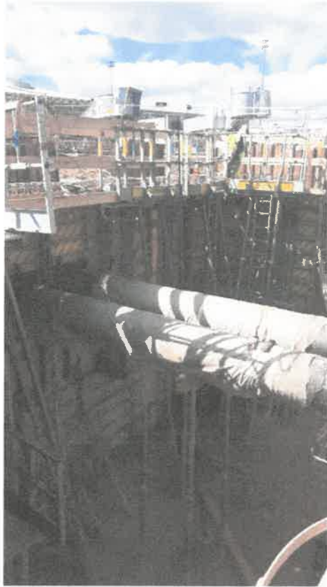
Construction of the valve room with existing jet-Fuel pipes
