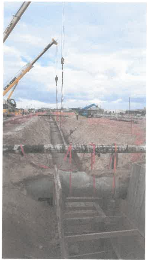
Pipelines laying
