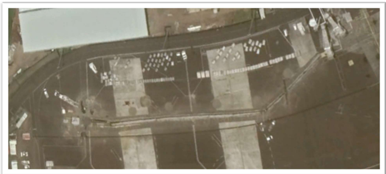
Aerial view of works
