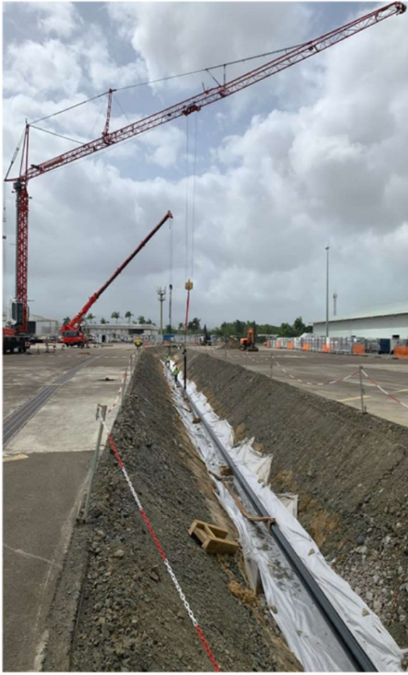
Pipeline lifting operations
