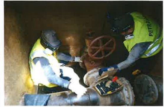
Installing a DBB valve in an operating hydrant system
